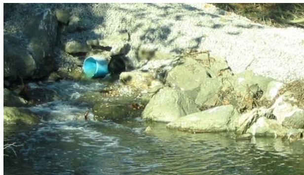
Bottom: One pipe and portion of gravel road used to cross to the far side of the dam. The excavators then work their way back across and remove the lowhead dam as they return to the starting point.
