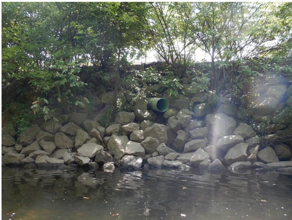
Photograph 4 (Taken 8/1/2019). Concrete slab armored bank with an outflow pipe that was not flowing during the sampling events. Photograph taken of stream bank left facing east.
