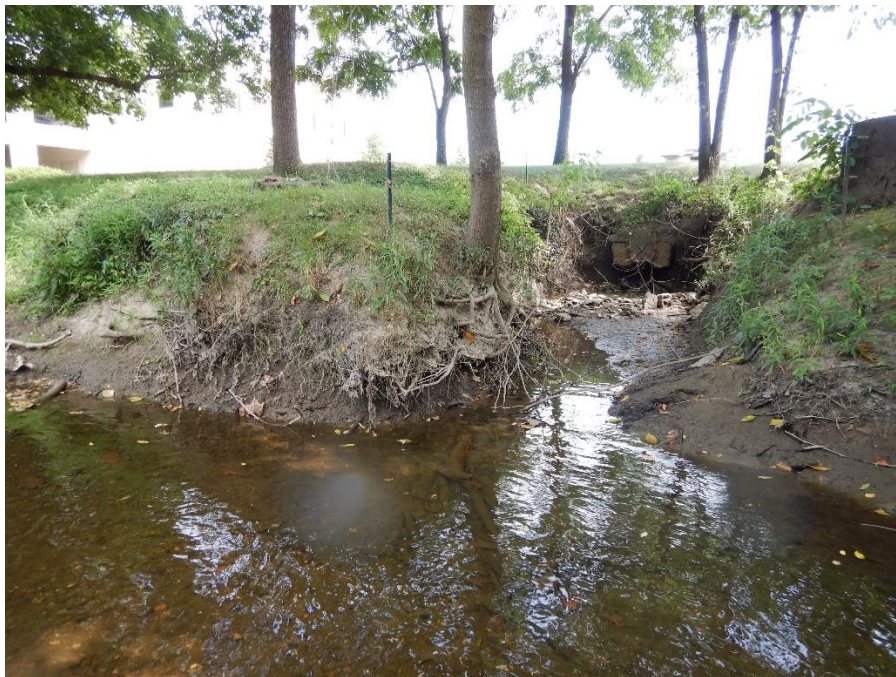
Photograph 6 (Taken 8/1/2019). A capped outflow culvert set back approximately 15 feet from Alum Creek was seen leaking liquid through the sampling events. Photograph taken facing northwest.
