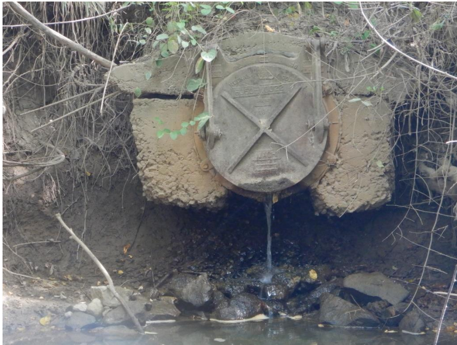
Photograph 7 (Taken 8/1/2019). Liquid seen flowing out of capped outfall pipe near the Industrial Site.
