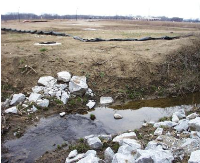
Figure 28: A failed sediment fence near an Alum Creek tributary allows sediment to wash into the stream.
